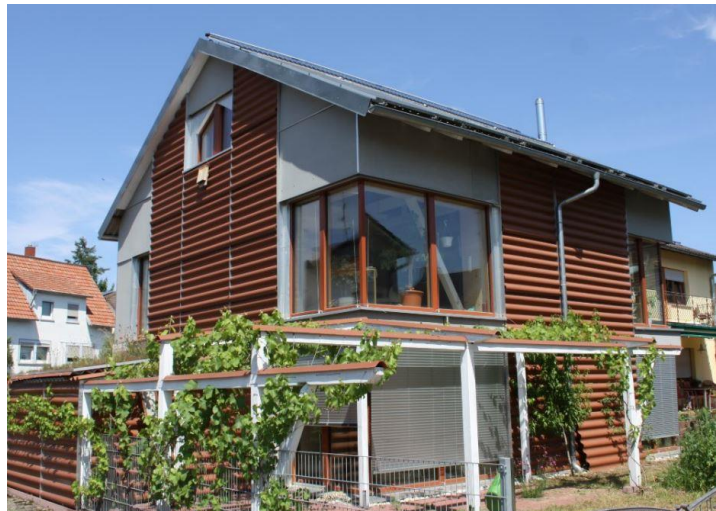
Loses little heat but gains a lot of it from the windows: in his Passive House, Benjamin Krick only has to use additional heating for three months, with the heating switched off for the rest of the year.
